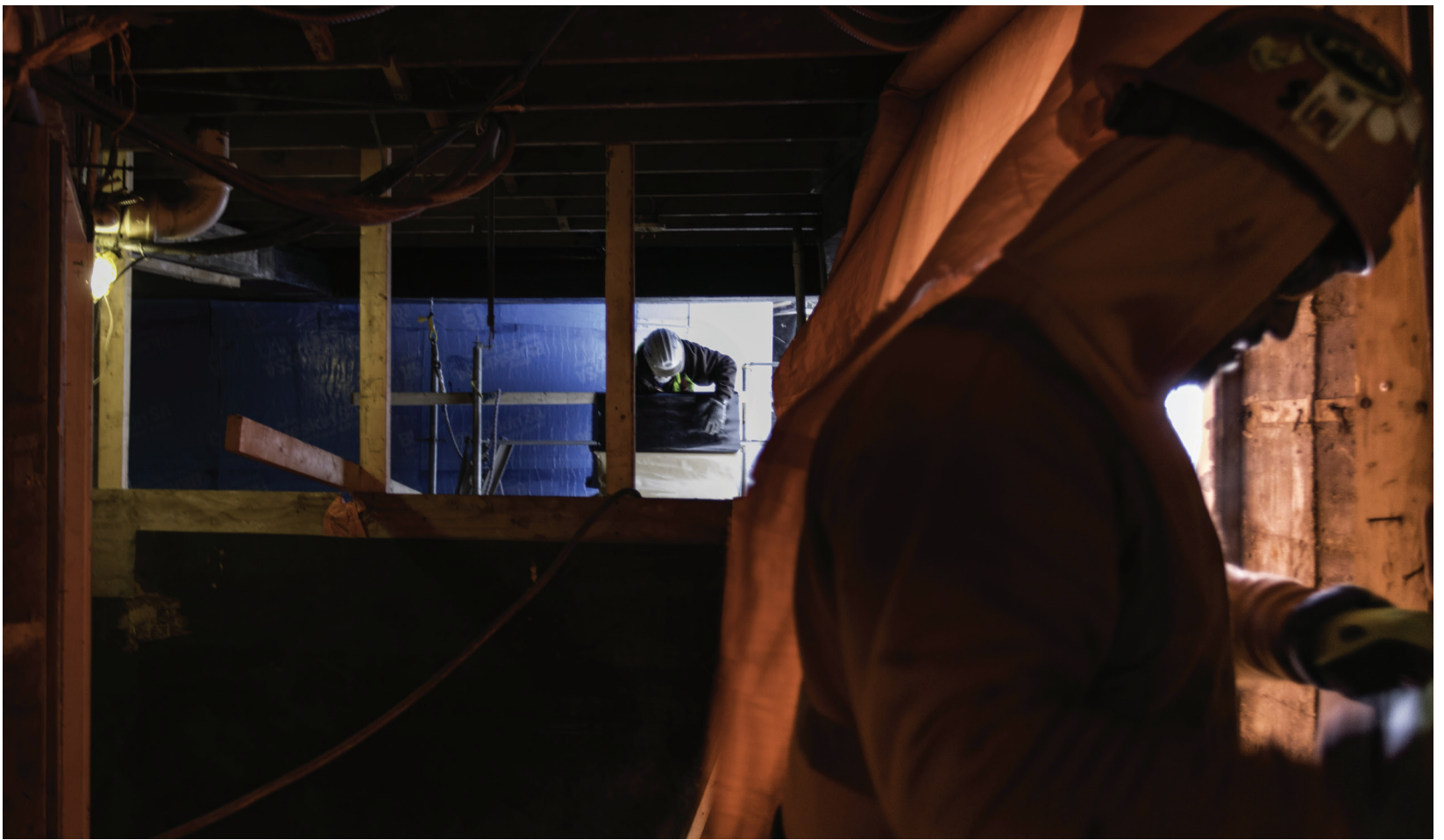
▲ Then and now: The crew from 1937 taking a break from working on the construction of our 1938 building (left). Above, our current crew is hard at work on the Atrium Space.
